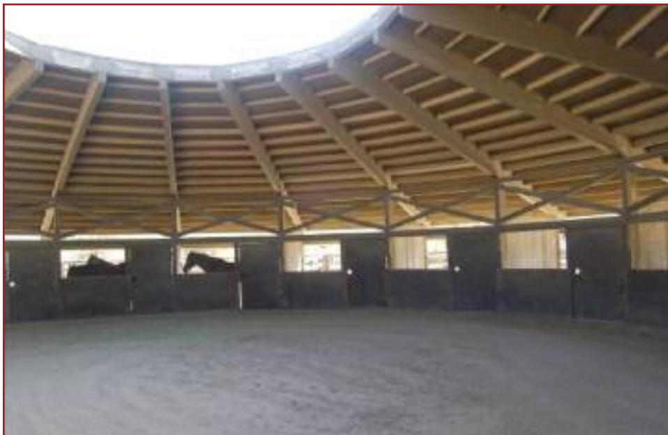
Inside View of Horse Barn
